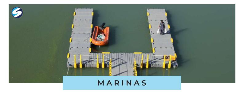
Marina is a floating dry dock, a floating pier. It can be used as a platform or ramp supported by pontoons. Marina is usually joined to the shore with the help of a gangway. The dock is controlled in place by vertical poles called pilings, which can be held together with the use of anchored cables.
